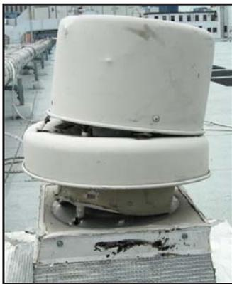
Wind damaged fan and cowling
