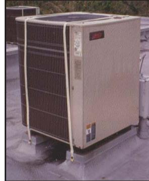
Well secured with straps, 2 screws desirable per strap connection
