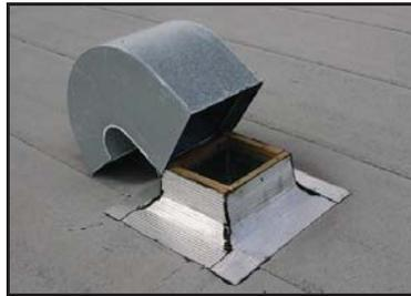
This goose-neck was secured with two screws.
