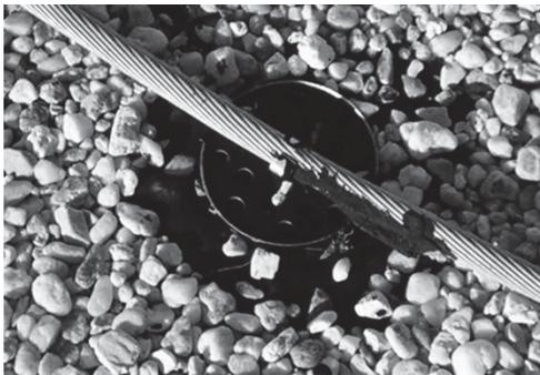
Conductor secured with clip adhered to cover
