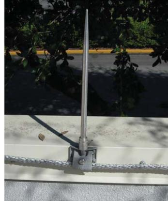
Air terminal screwed to wood nailer
