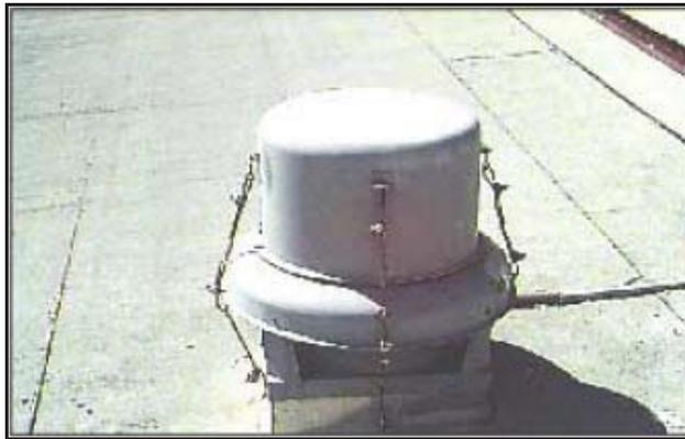
Secured fan and cowling
