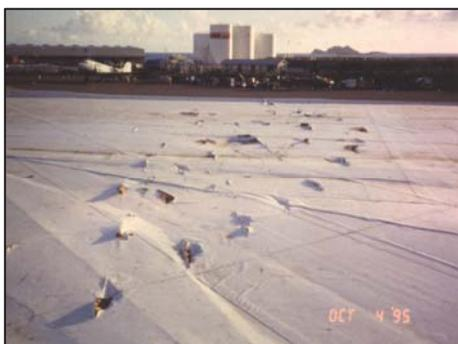
**Roof cover damage from equipment**
